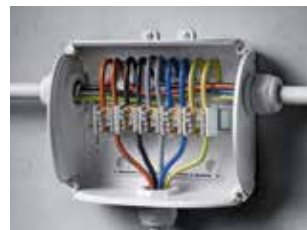
with Main line branch terminals
